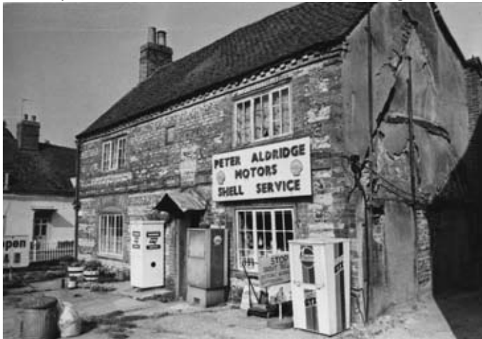
This is the one picture we have of that garage, looking a little worse for wear, taken perhaps just before it finally closed. Note however the easily visible cruck beams appearing from behind the cracking plaster.
