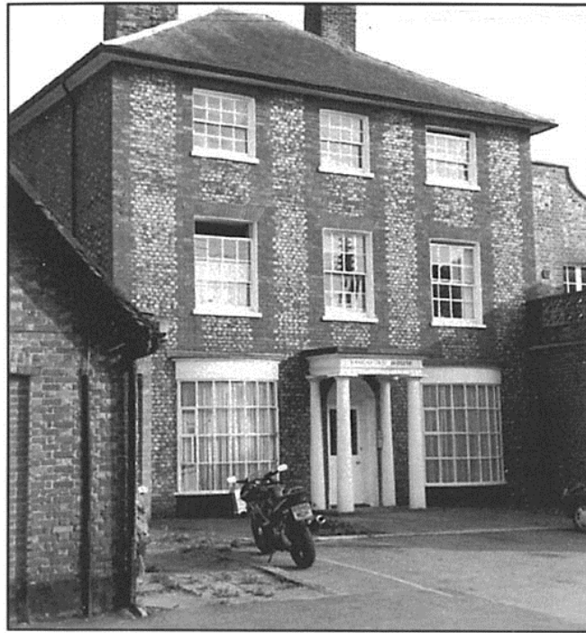
Fig 7.15: Kingsford house is an example of a new type of house, a villa, built in the early 19th century, and using blue/grey header bricks and red brick dressings to create the form of the facade
