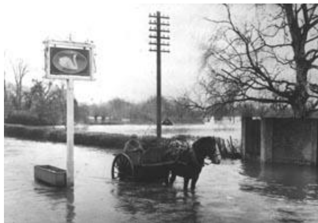
Floods at the Swan Public House
